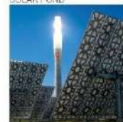
Gemasolar power plant in Spain
