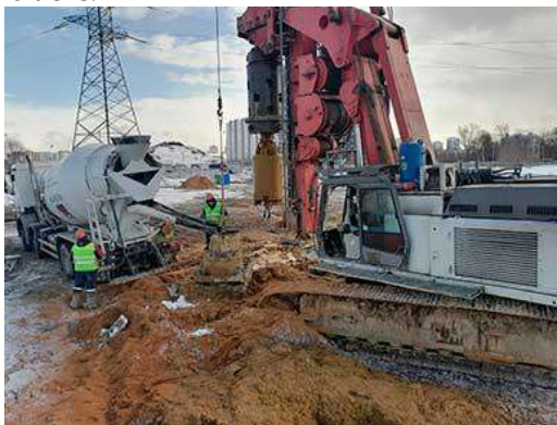
Fig. 6. Installation of bored piles using Double Rotary technology.
