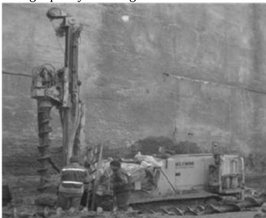
Fig. 2. Installation Klemm KR-70 for piling with short augers.
