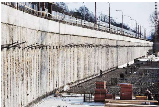
Fig. 1. Reinforcement of the pit walls with sheet piles with anchors.
