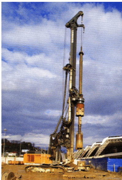
Fig. 5. Drilling rig JUNTAN PM-25.
