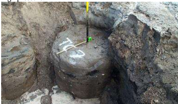
Fig. 1. Ground-cement piles.
