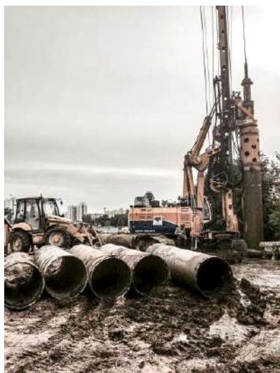
Fig. 7. Drilling wells under the protection of inventory pipes.
